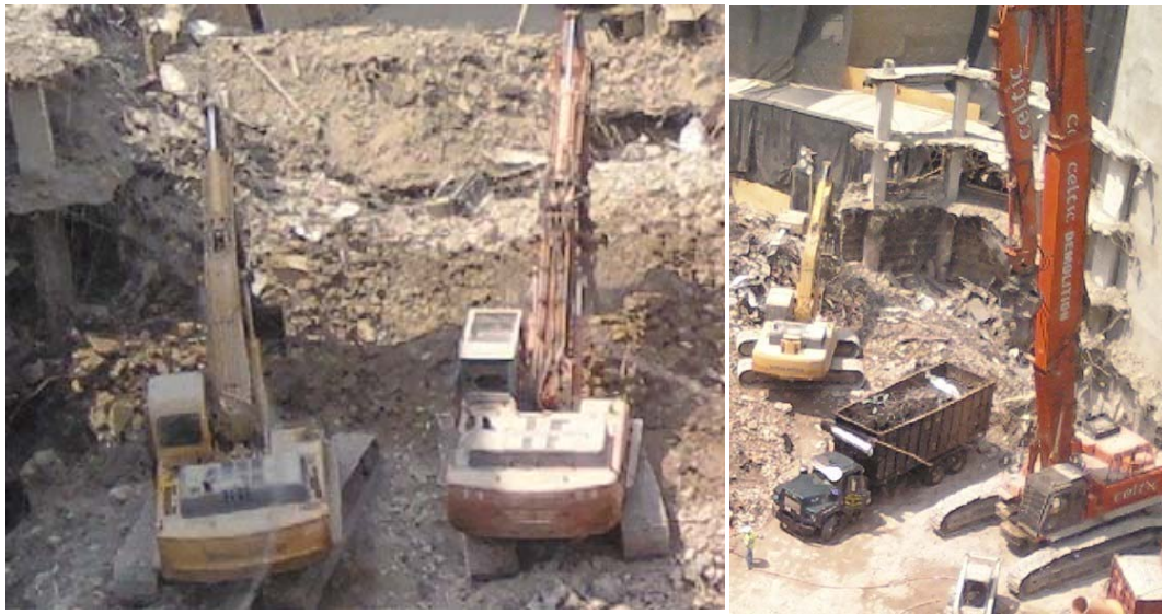
Figure 6- Excavators w/ hydraulic shears
