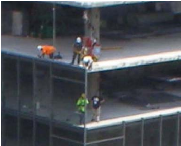
Figure 13 - Curtain Wall Being Hung at Lafayette Tower
