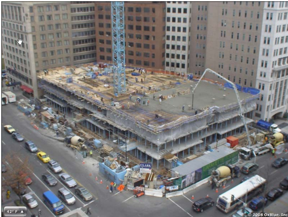
Figure 4 - Superstructure Site Picture
