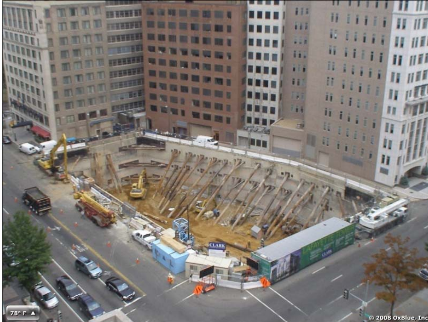
Figure 3 - Demolition Site Picture
